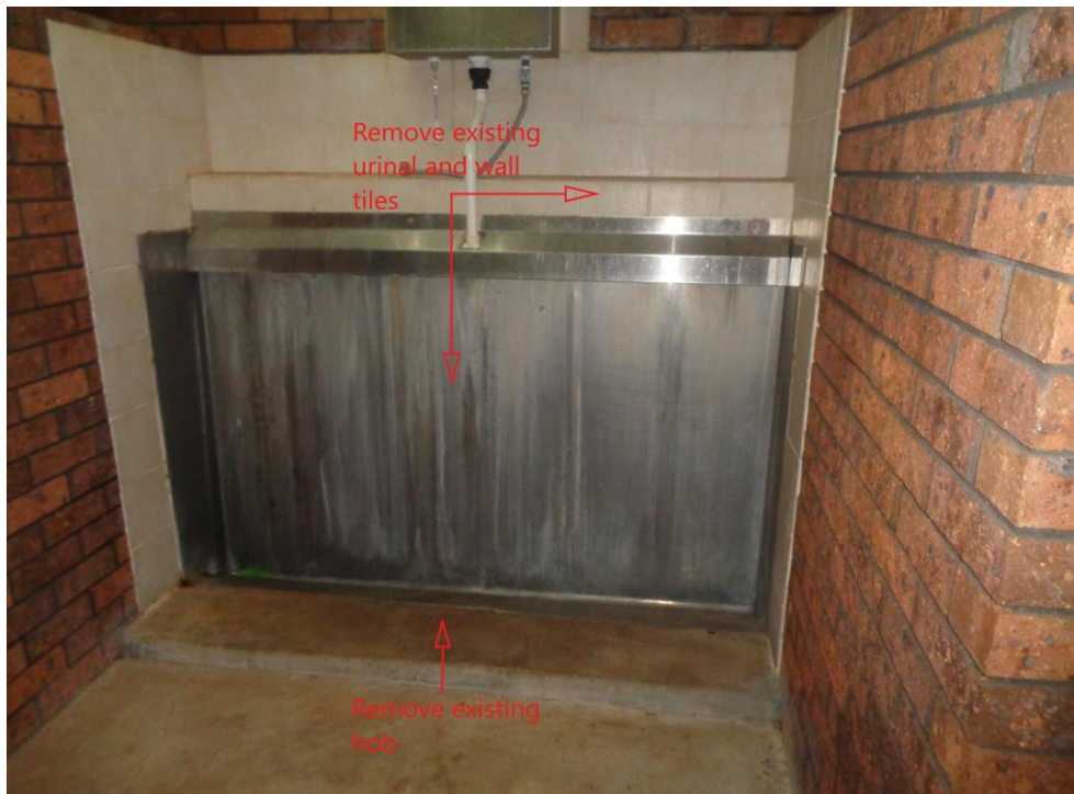
Figure 4: Demolish and remove existing urinal
