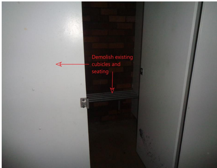
Figure 8. Demolish and remove existing changerooms and seating
