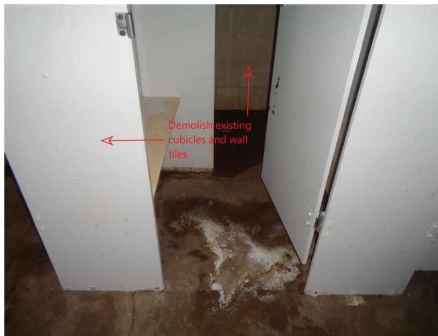
Figure 7. Demolish and remove existing shower cubicle walls
