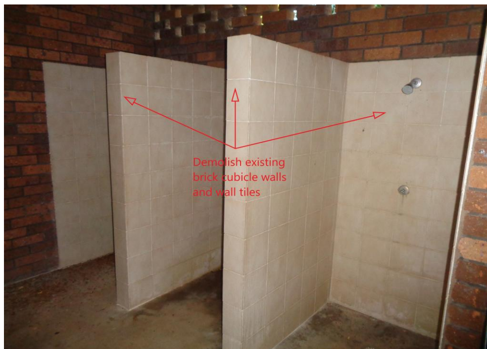
Figure 3: Demolish and remove existing cubicle walls
