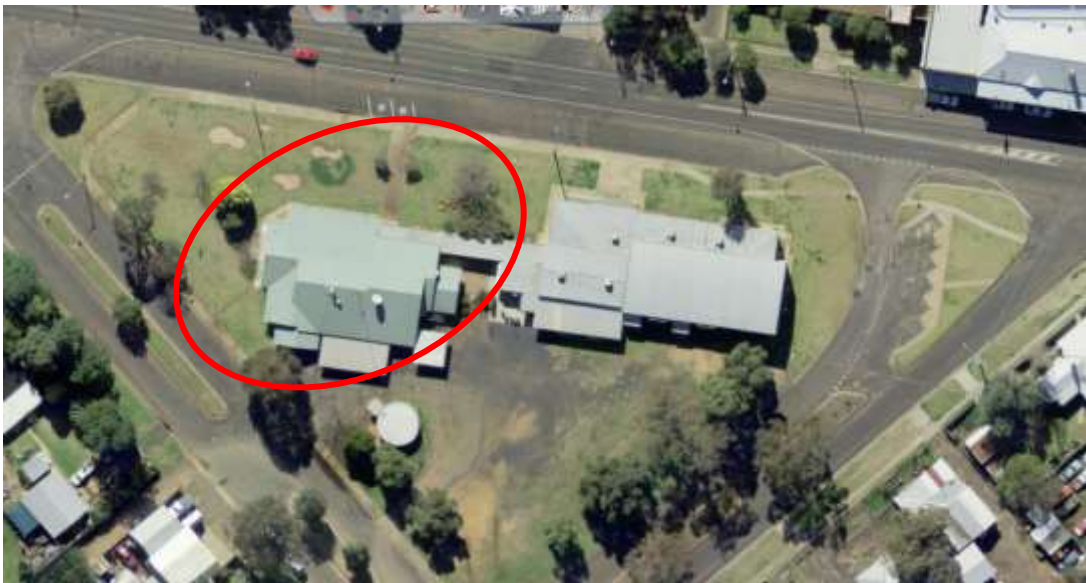
Figure 1: Gilgandra Shire Council building
