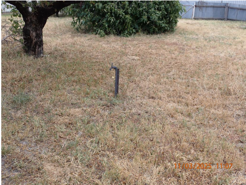
Figure 18: Stand pipe to be disconnected and removed
