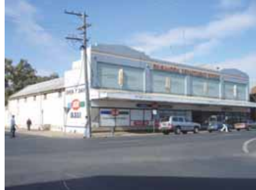
The former Western Stores on the corner
