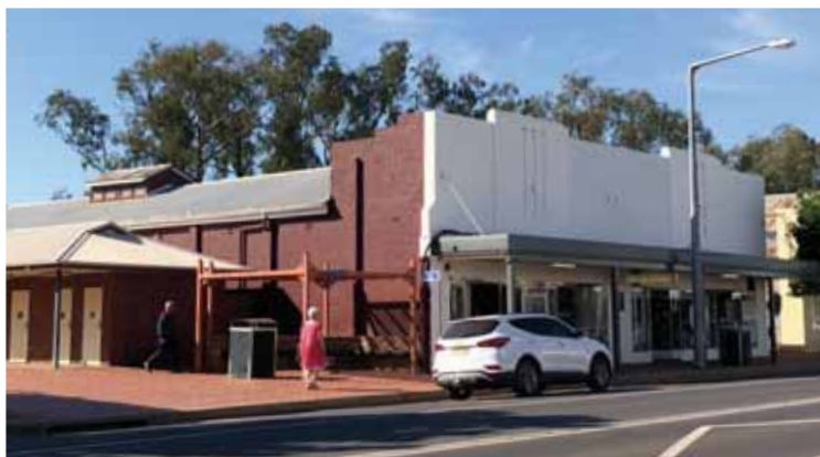
Existing building on 30-32 Miller St, December 2020.
