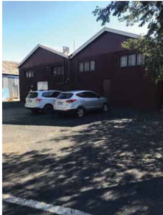
P8 – View of rear of future Library building. 2 or 3 cars normally park there.
