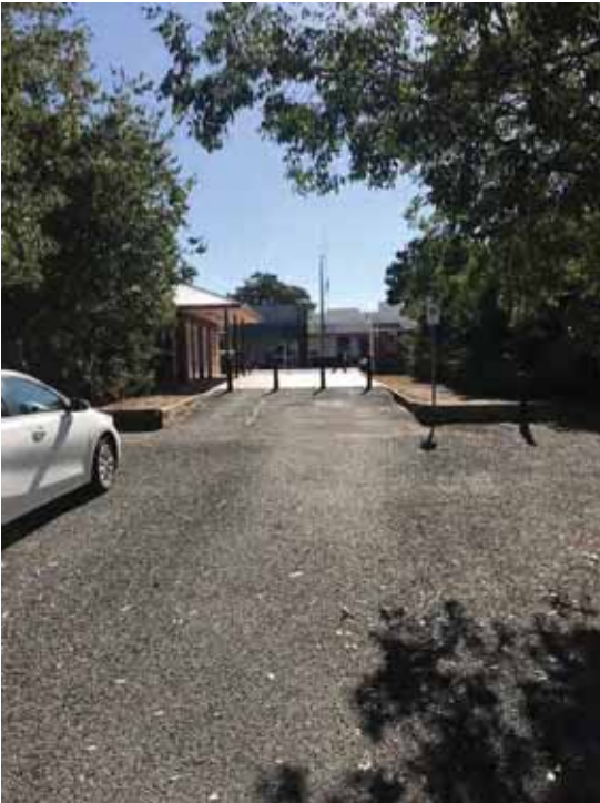
P10 – View of disabled parking space at rear of plaza from river parking.
