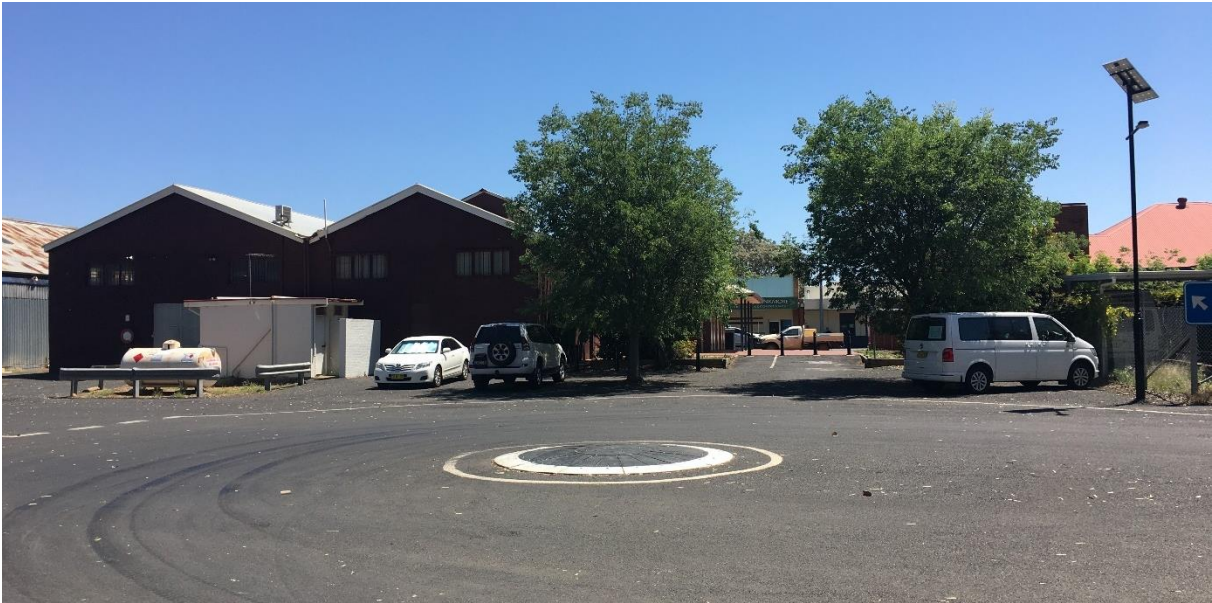
Figure 9: Rear of existing building and car park on subject site, viewed to north west
