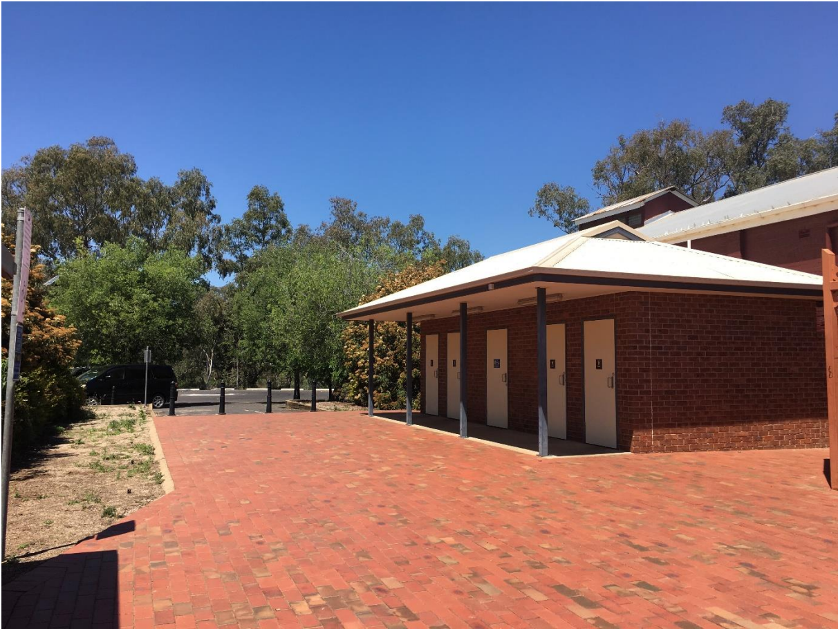
Figure 10: Existing plaza and amenities block on subject site, viewed to east
