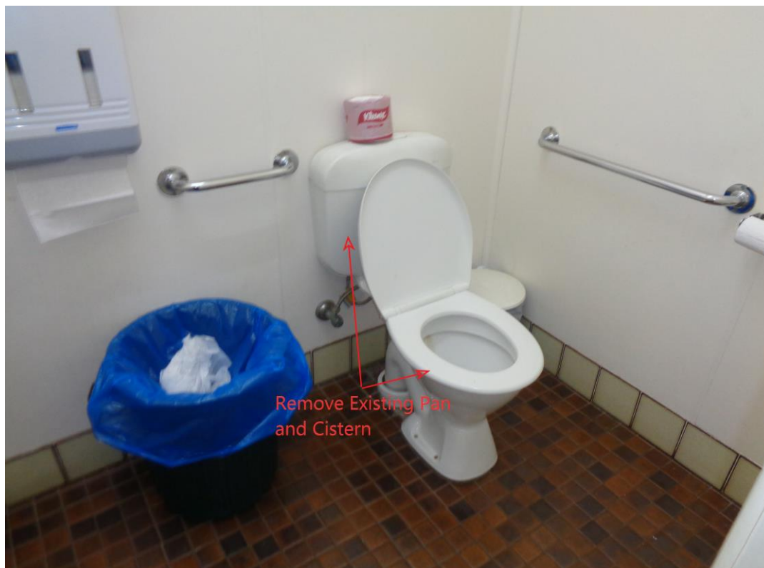
Figure 17. Demolish and remove existing pan and cistern
