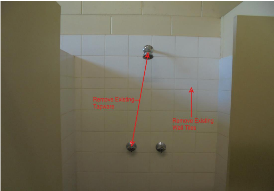
Figure 7b. Demolish and remove existing wall tiles and tapware
