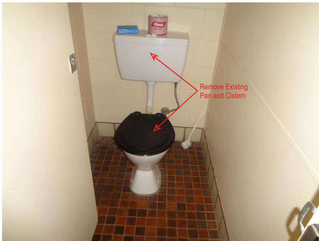
Figure 4. Demolish and remove existing pan and cistern
