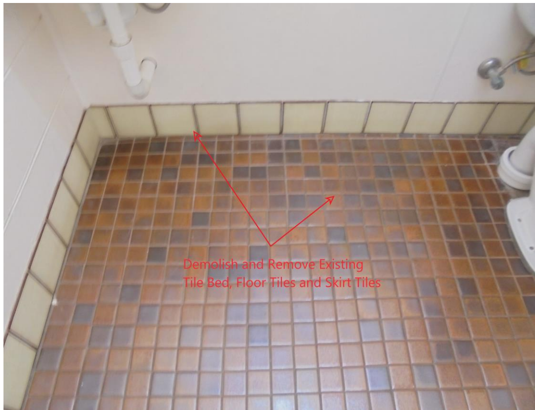
Figure 19. Demolish and remove existing tile bed, floor tiles and skirt tiles
