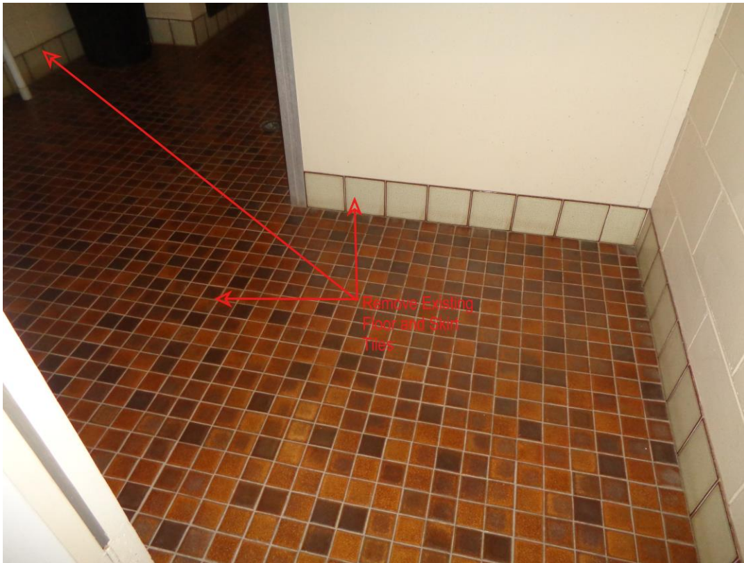
Figure 8. Demolish and remove existing floor and skirt tile
