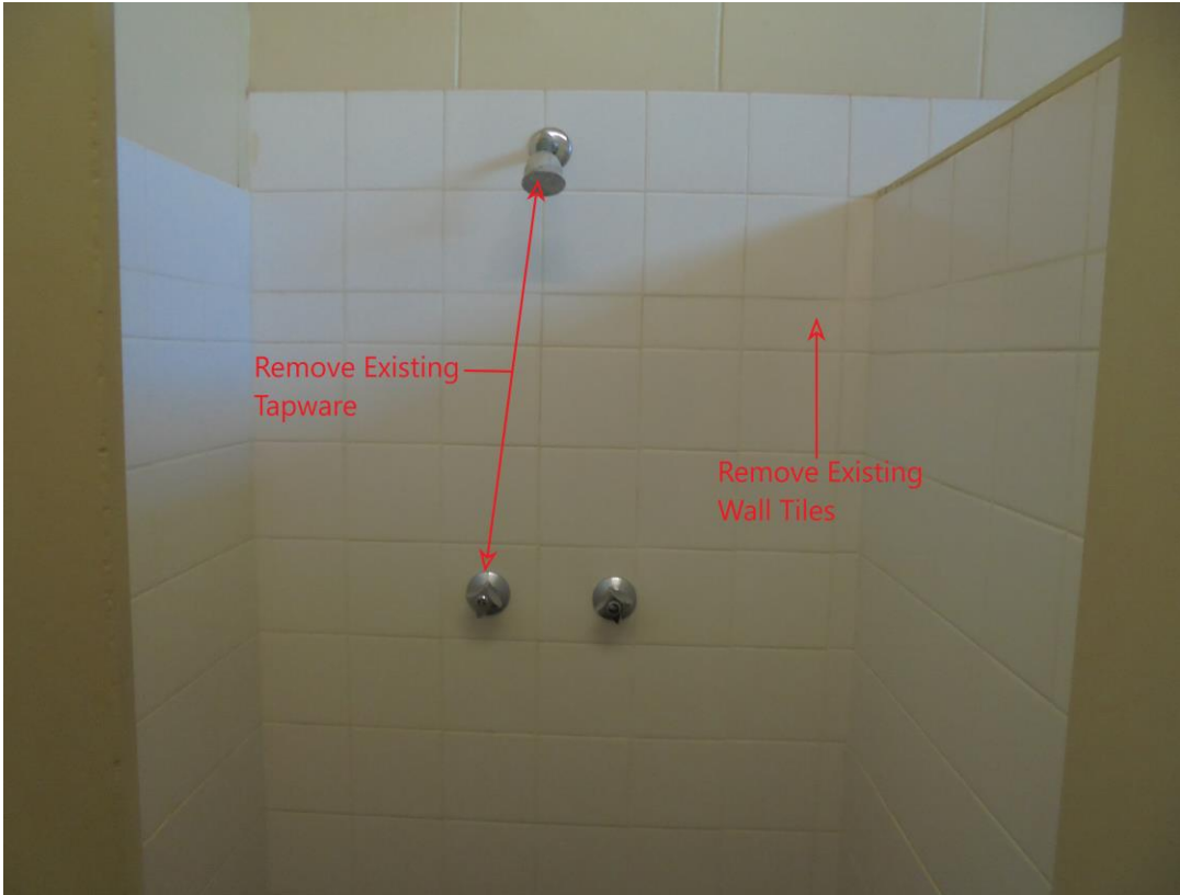
Figure 13b. Demolish and remove existing wall tiles and tapware
