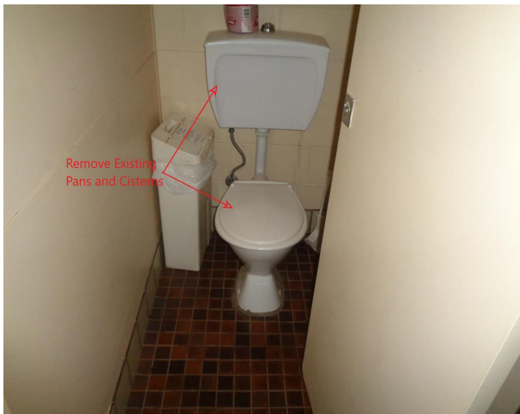
Figure 11. Demolish and remove existing pan and cistern.
