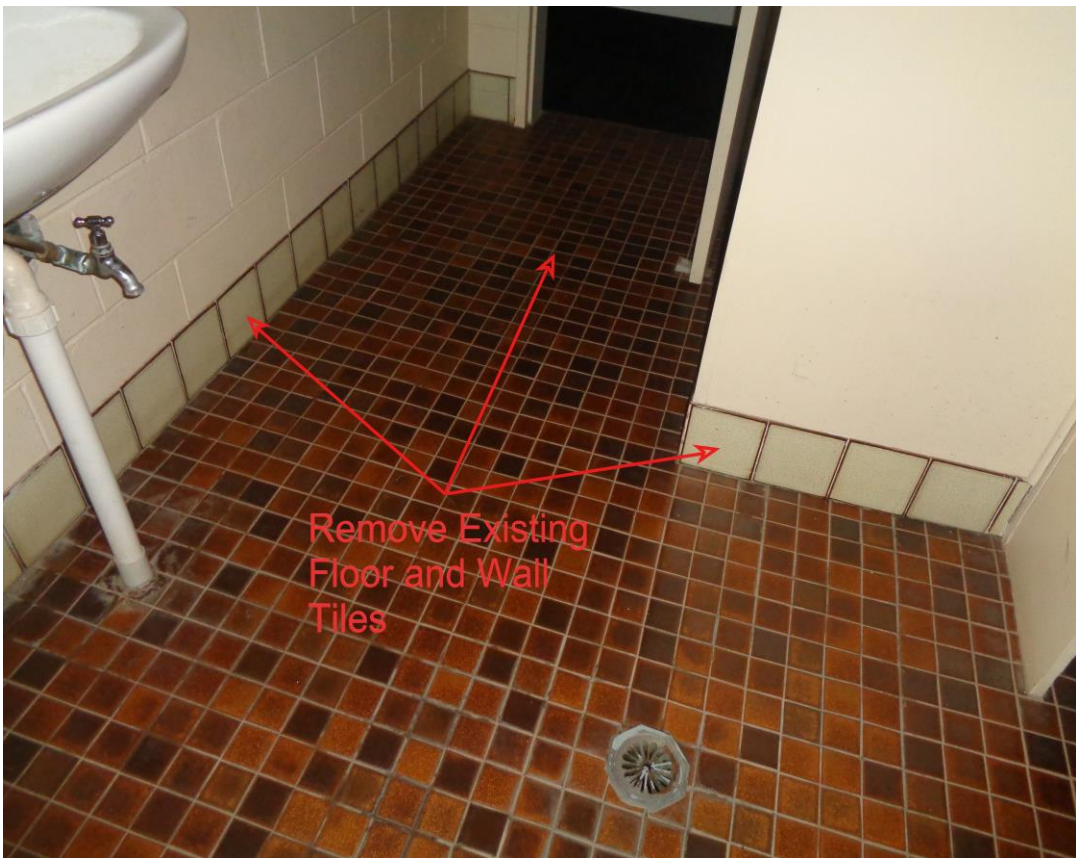
Figure 14. Demolish and remove existing floor and skirt tile
