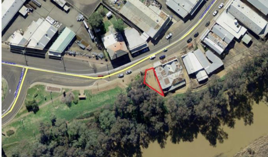
Figure 1 Site Location - Miller St next to Central Stores, Gilgandra
