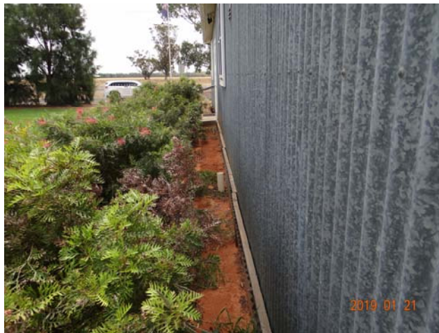
Figure 6 Reshape garden bed to allow ventilation under the building
