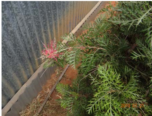
Figure 5 Remove loose corrugated iron to allow ventilation under the building
