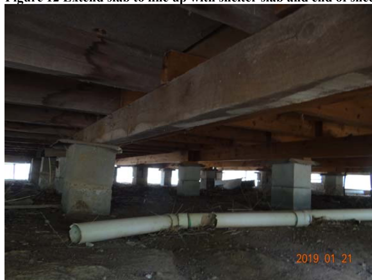
Figure 13 Existing structure beneath floor
