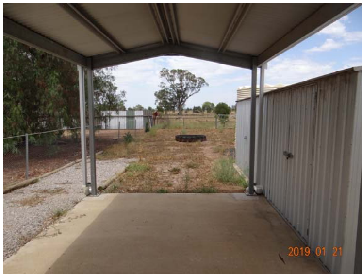
Figure 12 Extend slab to line up with shelter slab and end of shed
