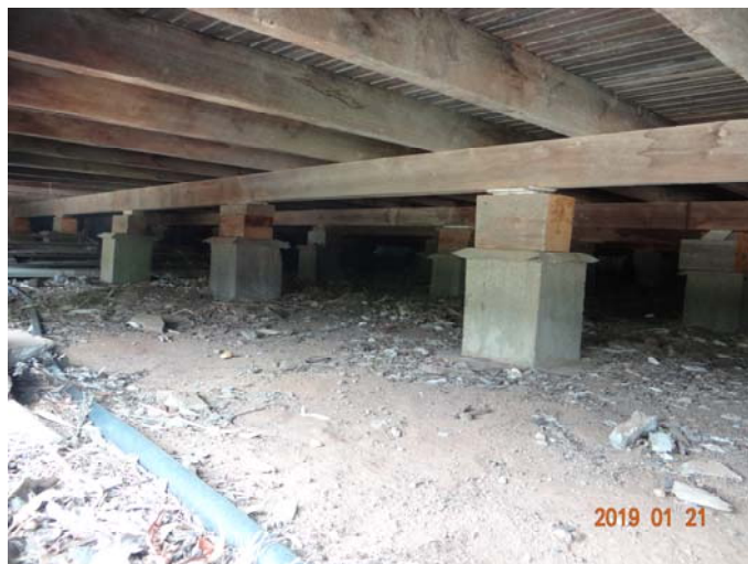
Figure 11 Existing footings under the hall
