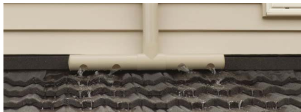
Figure 9 Example of stormwater drainage spreader
