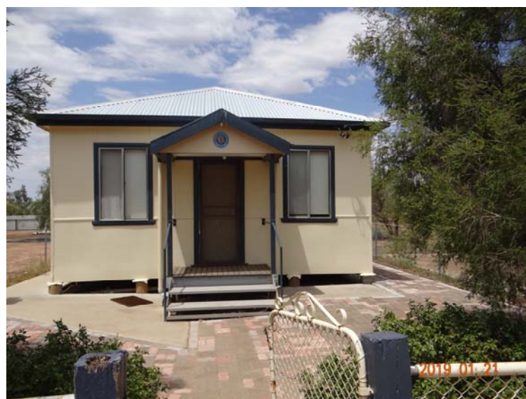
Figure 4 Front of Armatree CWA Hall
