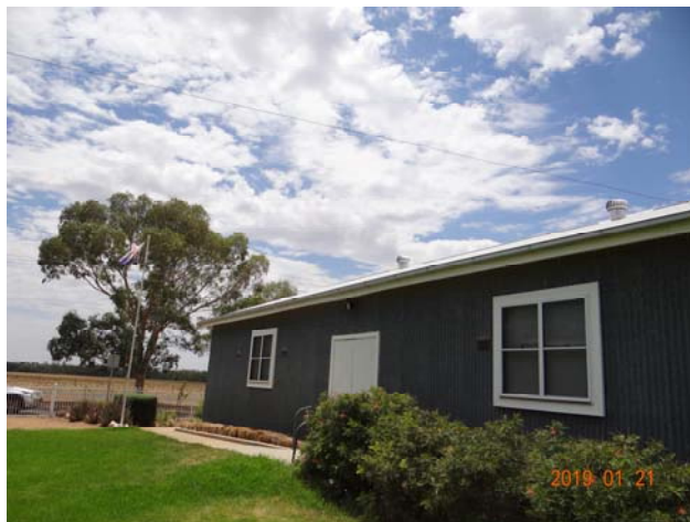
Figure 7 Run a new stormwater drainage line alongside the right-hand side of building with down pipes at 12m centres with adequate fall to drain into the water tank at rear of building.
