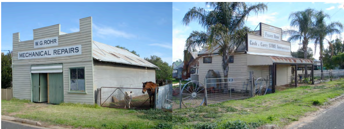
Plates 4.7 & 4.8: Tooraweenah's preserved timber-framed commercial buildings provide Gilgandra Shire with a unique heritage resource.
